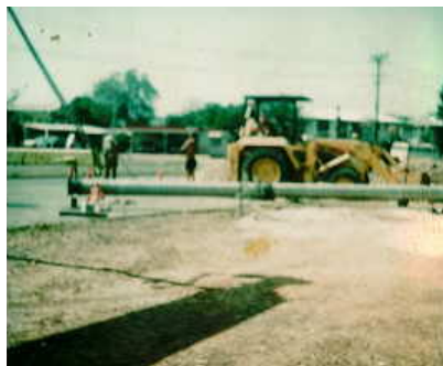
Coyder Road, 1979 – New MSCL Pipeline
